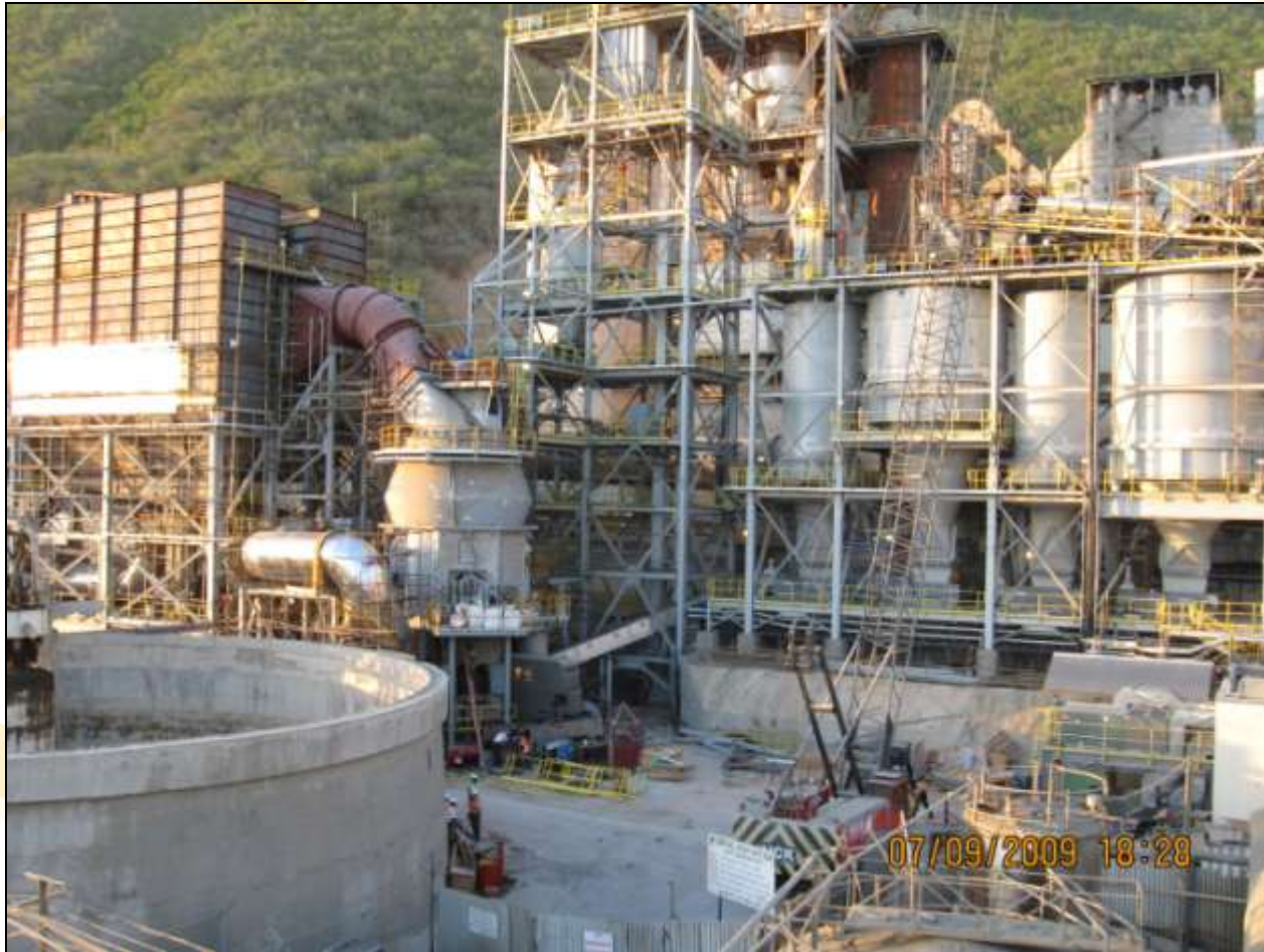
Overview of the entire Mill 5 Project at end construction
